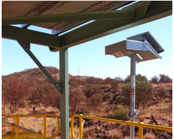
Boarding ramps and the SCL solar light with adjustable solar panel.
